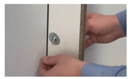
**Step 2**Thread 1 washer onto the screw and feed through the designated holes. Once through, add another washer and tighten in place with the wing nut.
