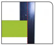
• Check the graphic panels are lined up with the centre line of the magnetic bar, if this overlaps by just a little it will give the appearance that part of the magnetic bar will not work
